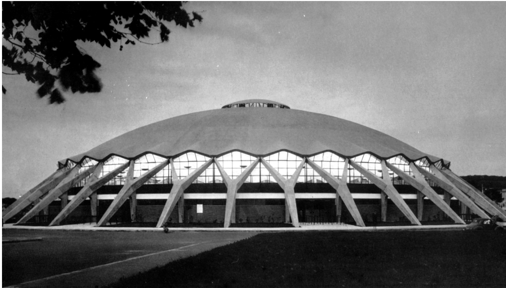
4. The Palazetto dello Sport, Rome, Rome. Pier Luigi Nervi, 1958. Exterior view showing forked columns. (From Pier Luigi Nervi, Buildings, Projects, Structures: 1953–1963 (New York: Praeger, 1963).)
