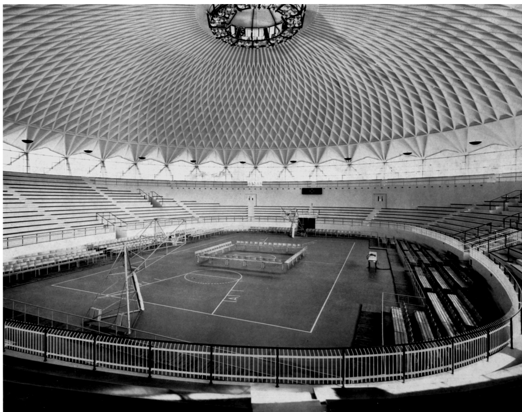
5. The Palazzetto dello Sport, Rome. Pier Luigi Nervi, 1958. Interior view showing pattern of concrete ribs. (From Pier Luigi Nervi, Buildings, Projects, Structures: 1953–1963 (New York: Praeger, 1963).)
